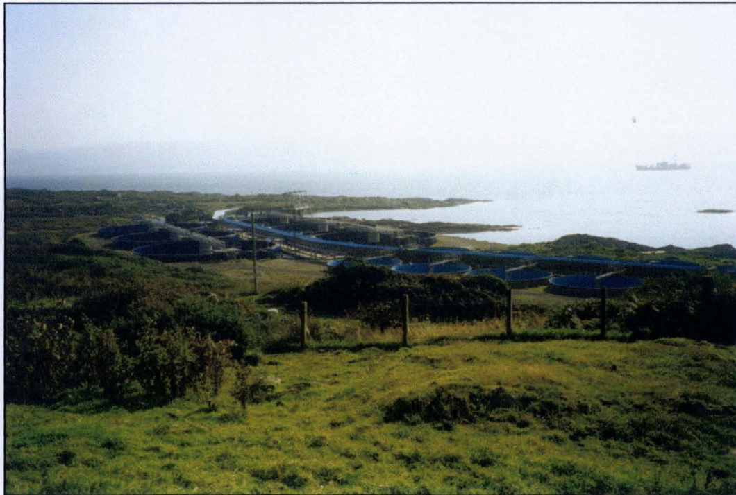
Figure 2.1.13 View of a large pump ashore facility on the west coast of Scotland showing an open distribution channel running between the tanks.
