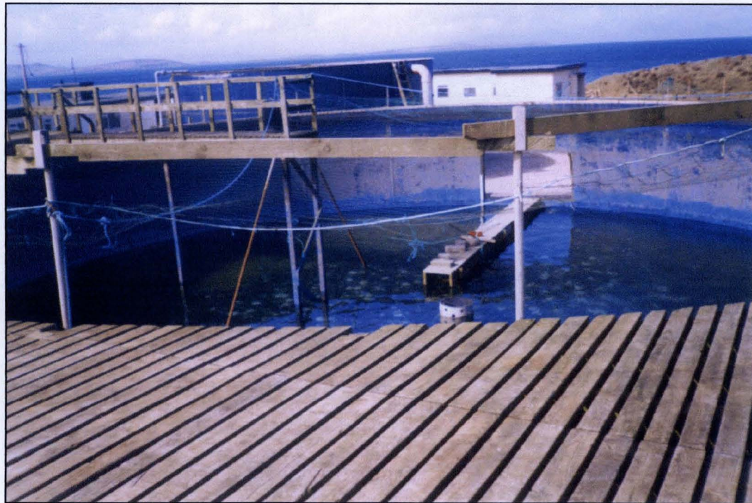
Figure 2.1.15 View of a large 24m-diameter, shallow circular tank with a central drain, adapted for turbot having previously been used for salmon
