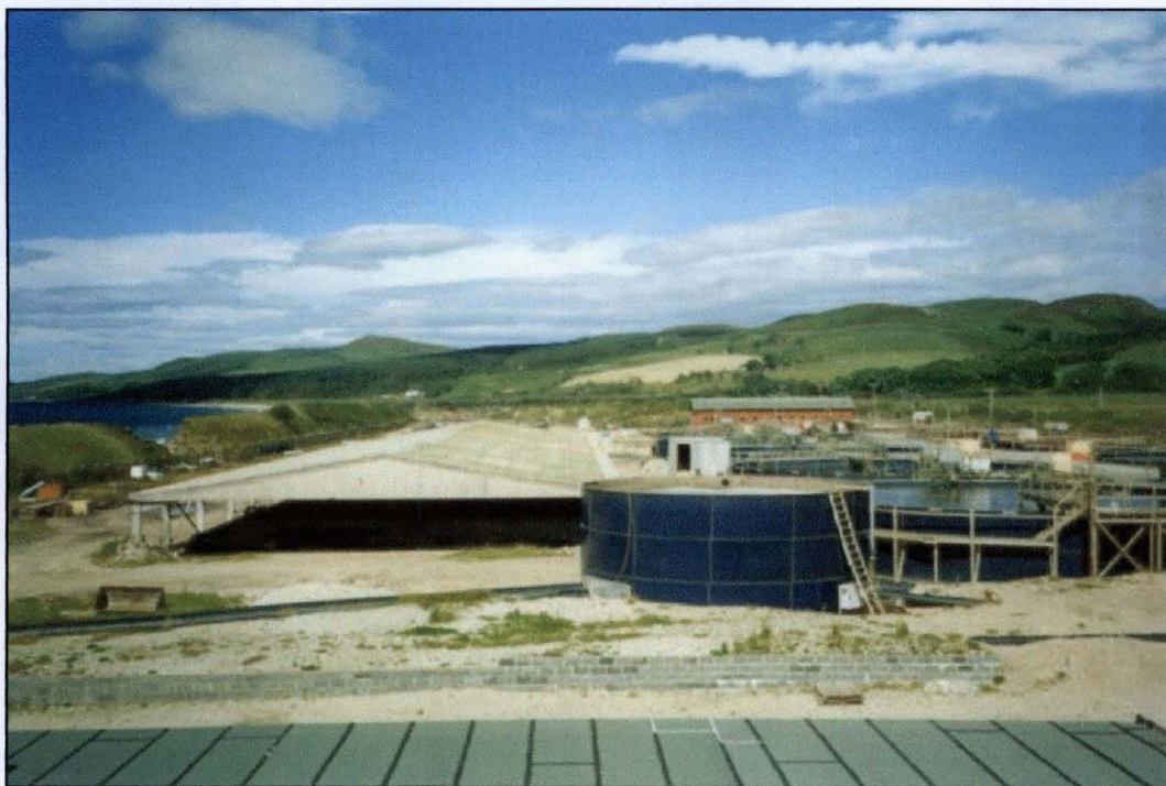
Figure 2.1.12 View of a large flow through facility (tanks and raceways) on the west coast of Scotland used for both salmon and turbot. The large blue tank in the foreground is one of two header tanks supplying the rearing tanks.
