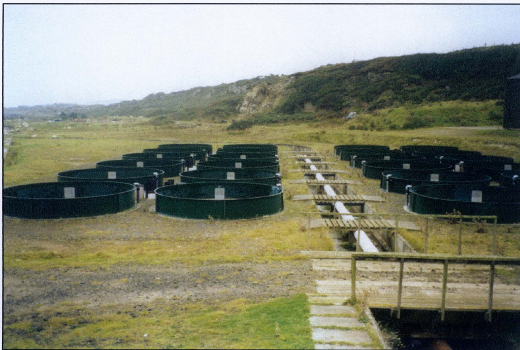
Figure 2.1.14 View of a pump ashore facility in Scotland showing the water distribution pipe running centrally between the circular 5m diameter tanks.
