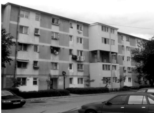
Low-comfort blocks: attaching new balconies
