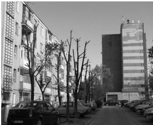
The 1960s: Blocks in masonry and in situ concrete shell
