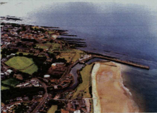
Plate 6.9: Lack of Sediment North of the Harbour
