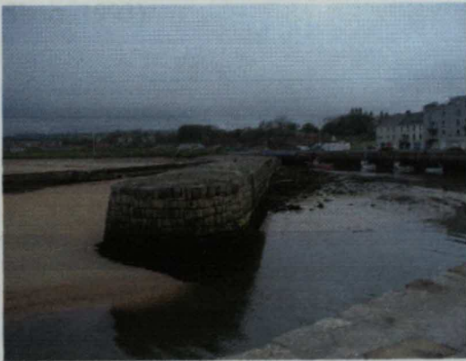
Plate 6.8: Sediment Piled at end of Cross Pier/Harbour Mouth
