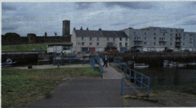
Plate 3.14: Footbridge and with attached Sluice Gates
