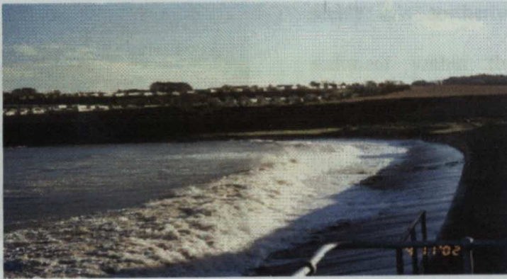
Plate 6.5: Surging Breakers, inundating right to the Central Seawall
