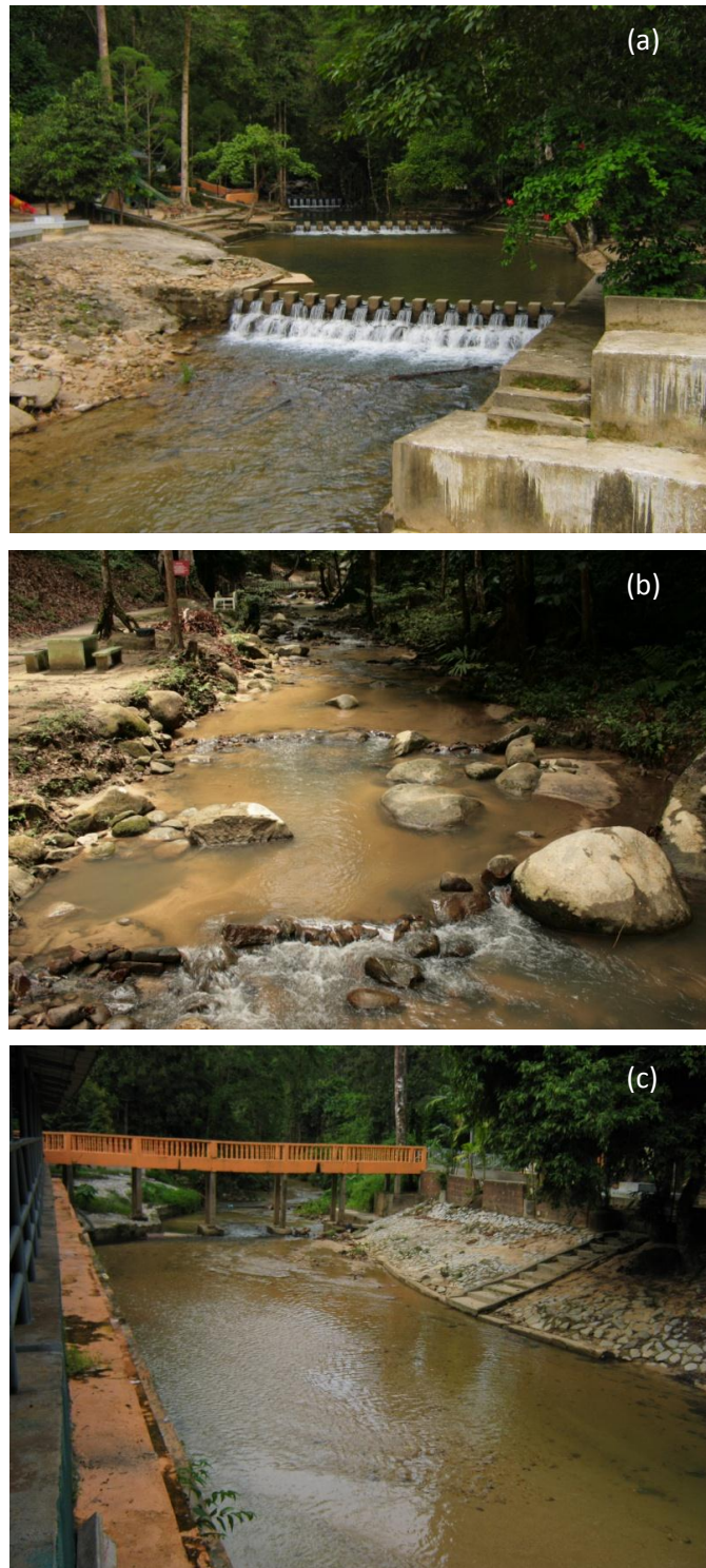
Figure 4.1. Profound small-scale habitat modification in small lowland streams in Peninsular Malaysia, a. Creation of permanent recreational pools in rapidly-flowing stream sections, b. Temporary pools along the stream section and c. Stabilisation or strengthening of the banks from erosions.
