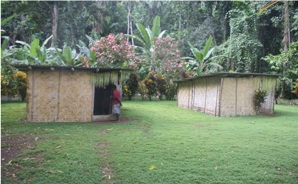
Figure 10. The Gavman Haus on the left and the Misin Haus on the right.
