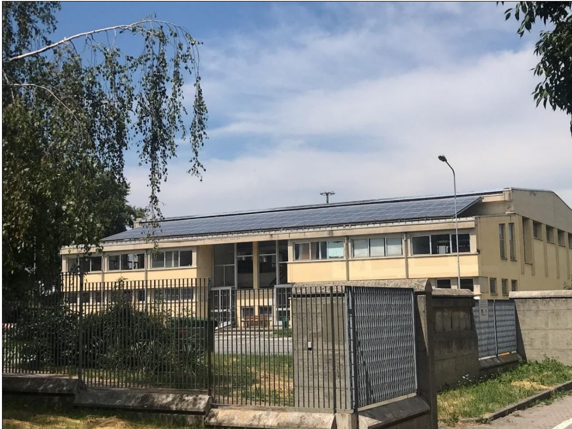
Figure 8. 50KWp solar facility on the roof of a high school in Cuneo, Piedmont. Established in 2010, the project was one of the several rooftop solar projects promoted by Solare Collettivo.
