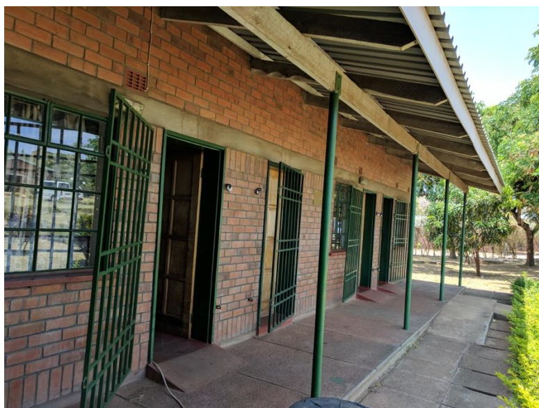
Figure 7: Ramps leading up to a school building and into classrooms.
