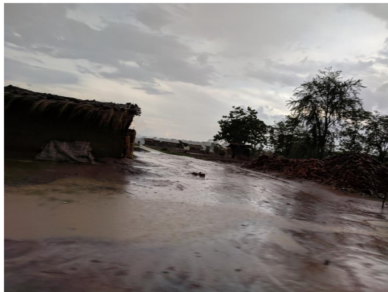
Figure 5: Roads beginning to flood during a storm early in the 2018-2019 rainy season.
