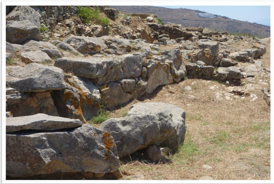
Figure 4.102 Cyclopean wall section at western end of fortification wall.
