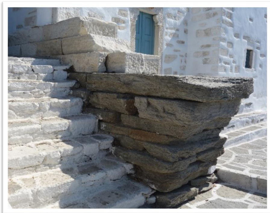
Figure 4.48 Archaic period Temple to Athena Foundations, schist under with marble over, Paroikia.
