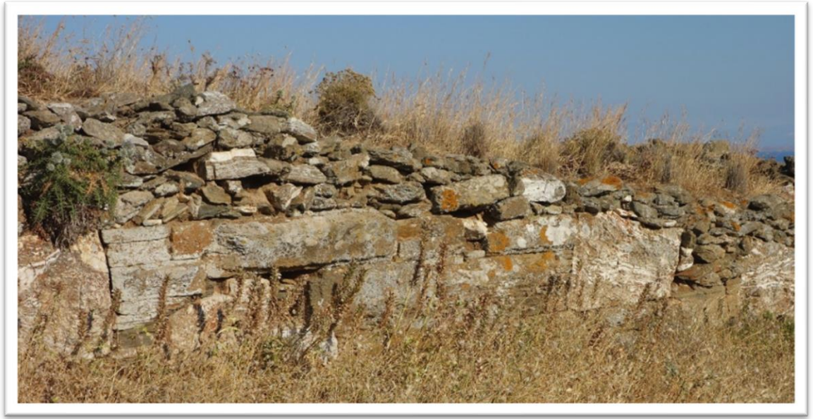
Figure 4.114 Wall section on westside of unexcavated acropolis.
