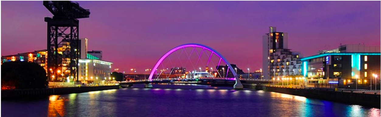
Figure 4.3. Clyde Arc, Glasgow.
