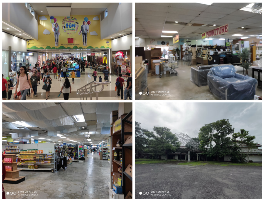
Figure 1: Top left—new lifestyle mall in Clark Freeport Zone. Bottom right—derelict duty-free mall in the same area and inside an open duty-free mall with visible structural issues (photographs by Lauren Crabb).
