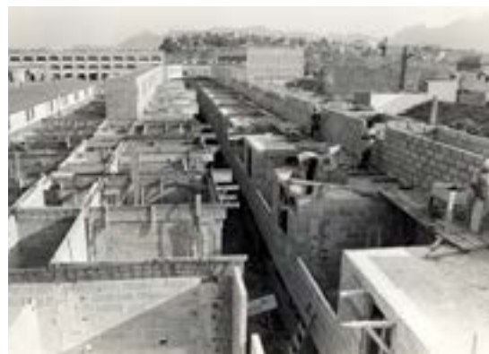
Figures 14, 15, 16. The construction of a new part of Nova Holanda, 1991.
