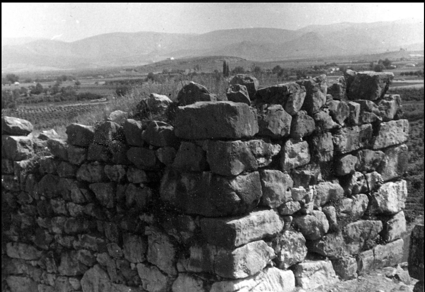
Tiryns, remains of the city walls.
