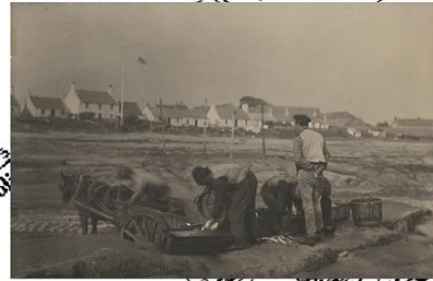
Work on the beach
