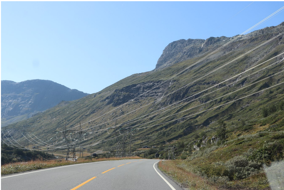
Figure 20. Power cables and masts bringing electricity from a hydroelectric dam to Oslo. Location: Hardangervidda, ca. 4hr. car-ride away from Oslo. Photograph taken by author.
