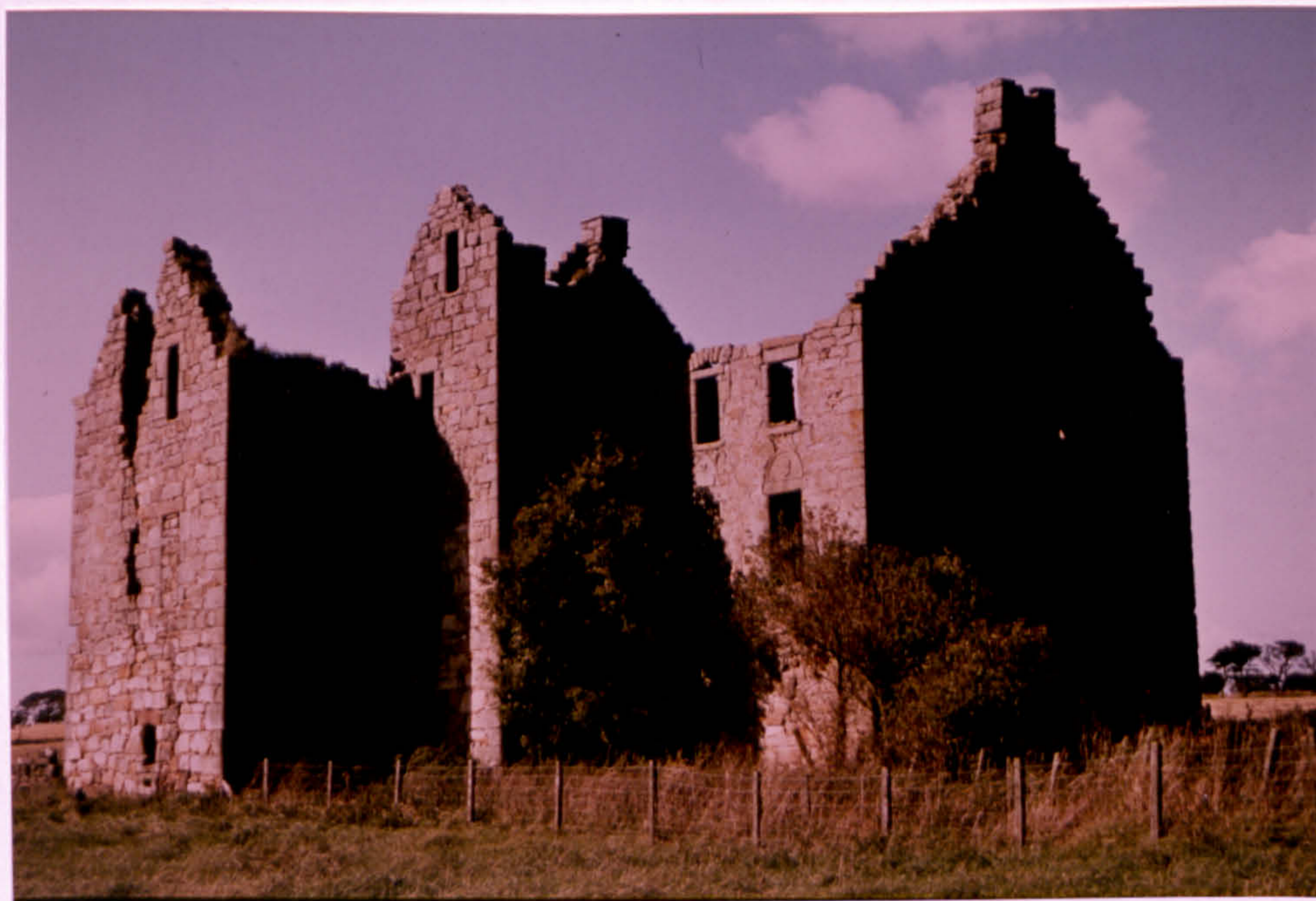
Plate 12.2 Pittarthie tower house from the south east
