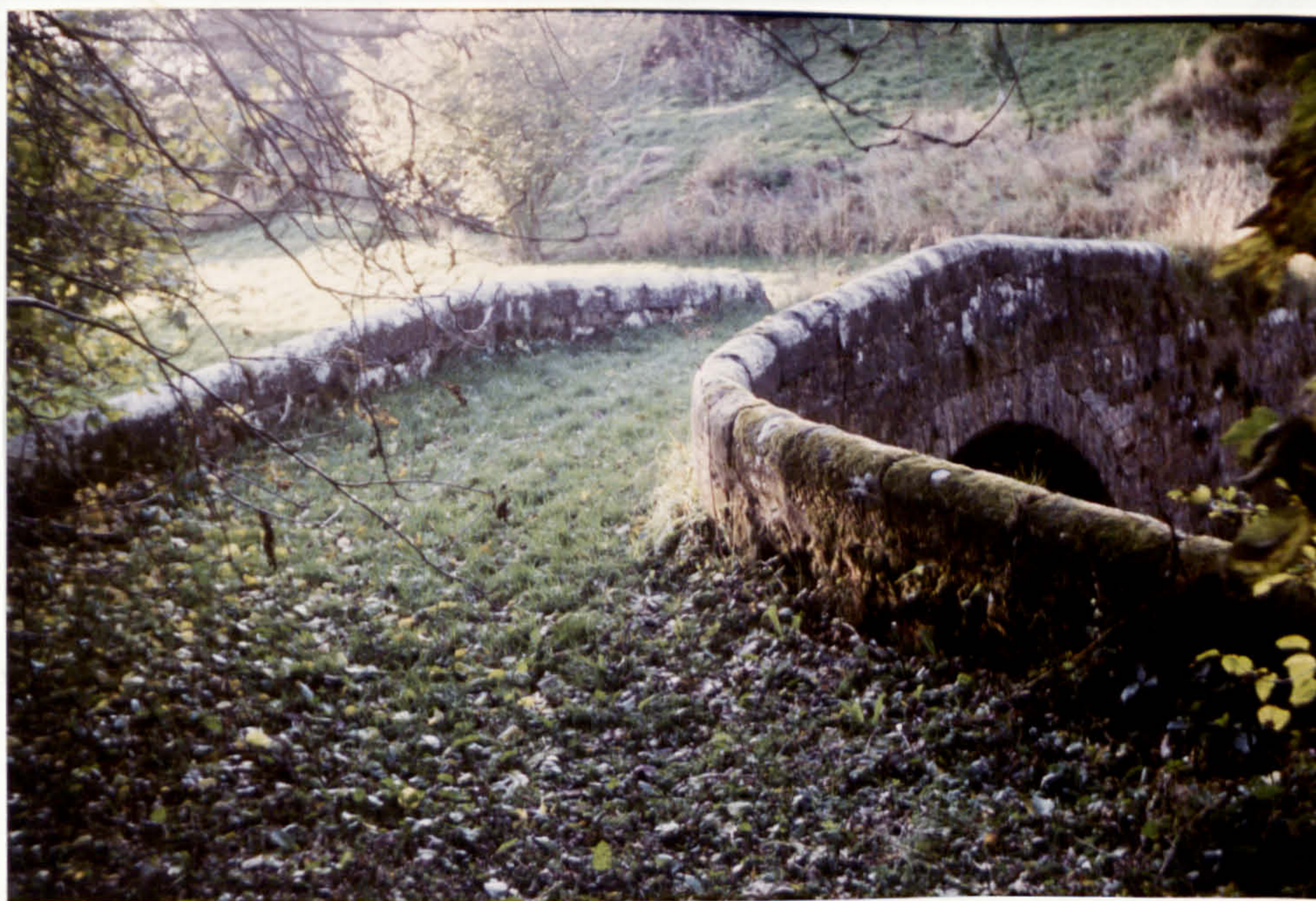
Plate 12.8 Peekie Bridge from the south east
