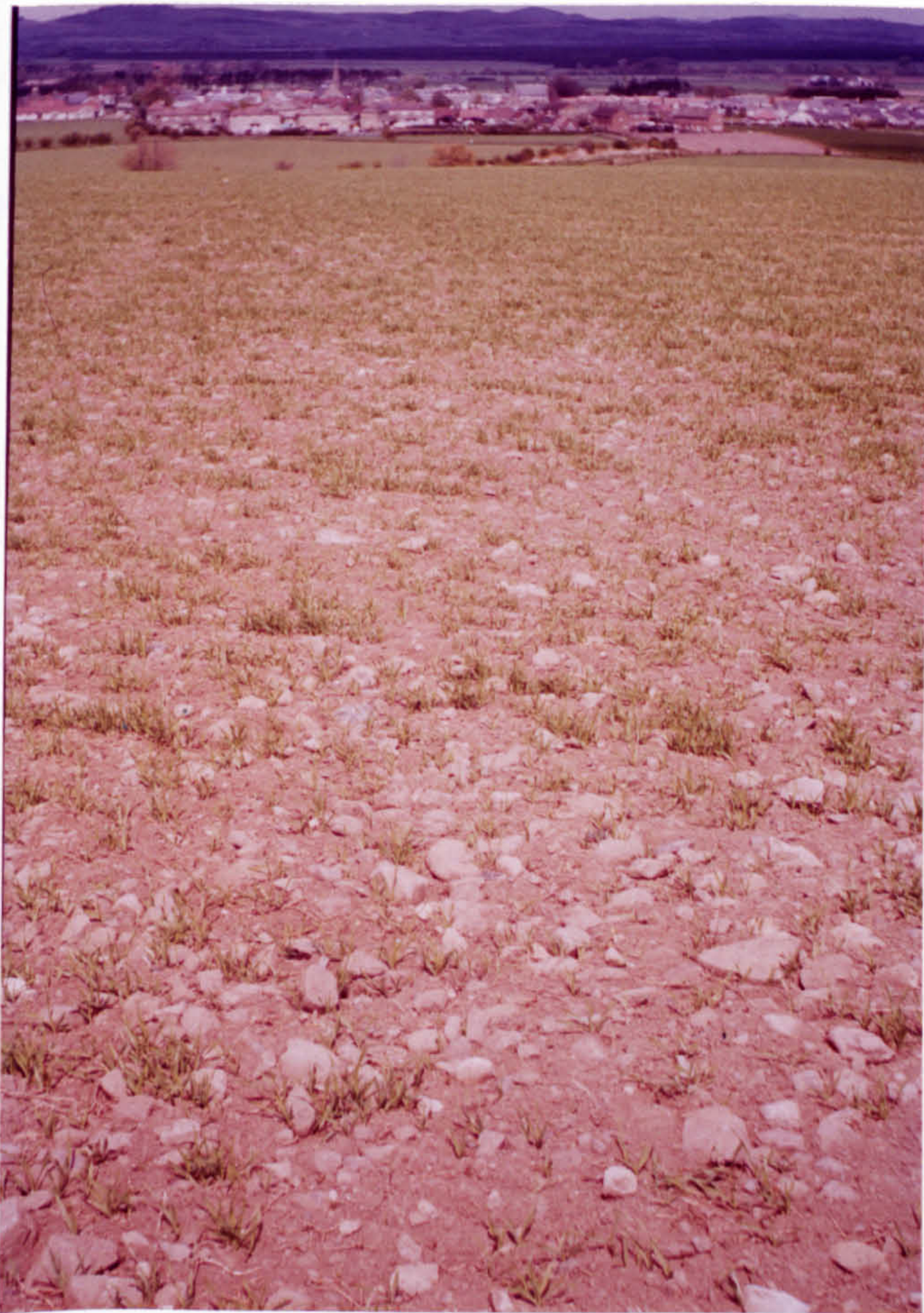
Plate 7.2 The old Shiels Bridge road: metalling A band of stones, size up to 15 cm, connects the bridge of Plate 7.1 to the surviving grass covered road leading into Freuchie.
