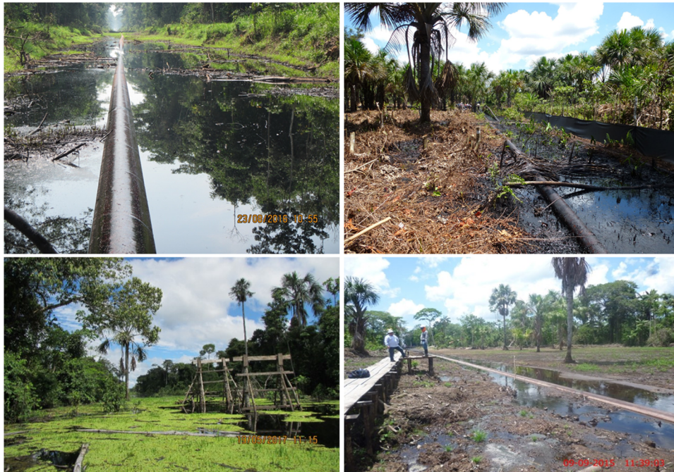
Figure 5. Oil infrastructure and contamination in the wetlands and peatlands of the Pastaza-Marañón Basin in Peru. Top left: dredged channel showing an oil pipeline during low river level. Bottom left: an oil spill at Lot 8 inside the Pacaya Samiria Nature Reserve, 2013. Right: remediation of a November 2014 oil spill near Cuninico showing the clearance of peatland vegetation during periods of (top) high and (bottom) low river levels. Source: All OSINFOR (InfraAmazonia 2021) except bottom left, ACODECOSPAT (2019).
