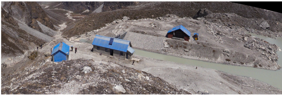
Fig. 14. Tsho Rolpa Spillway panorama (“© Reynolds International Ltd, 2016”).
