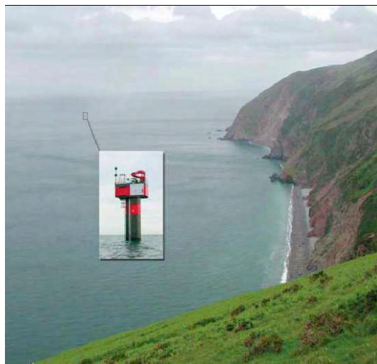
Figure 4.1 A photograph of Marine Current Turbine's Seaflow installation at Lynmouth, demonstrating the low visual impact of a single surface-piercing tidal stream device [62]
