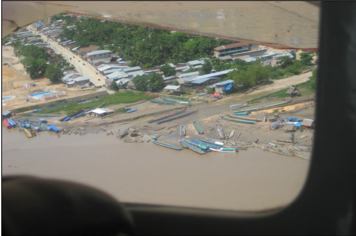
AN AERIAL VIEW OF THE MARKET PORT (DRY SEASON) AS I LEFT ATALAYA FOR THE LAST TIME. THE LONG GREEN BUILDING WITH A RUSTY ROOF TO THE RIGHT IS OIRA.
