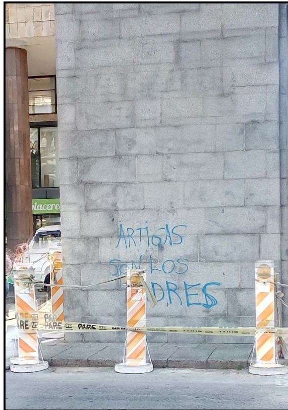
Figure 9 Graffiti on the Puerta de la Ciudadela on 4 November 2016.
