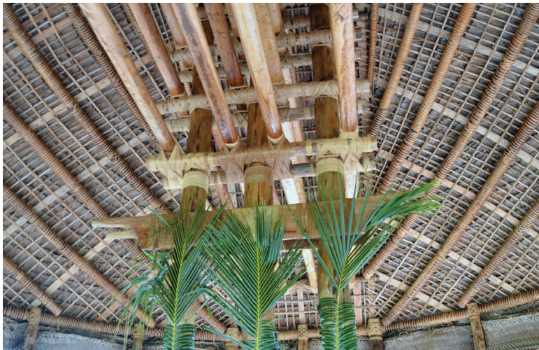
Figure 7.2: ’Afa binding on the roof structures in the fale at the Tiapapata Art Centre, Apia, 2014. Photo: Steven Percival.
