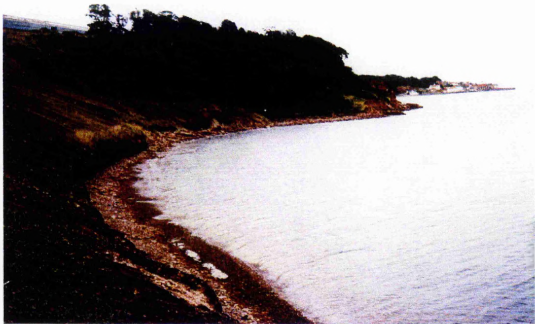
Plate 2.31 The Franceses beach looking towards West Wemyss (1992). The Franceses beach has been retained with strong mesh in an attempt to prevent any further erosion and the transfer of the material down coast.
