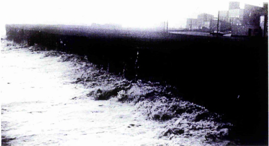
Plate 2.17 The erosion at Shore Street, Buckhaven, in 1974.
