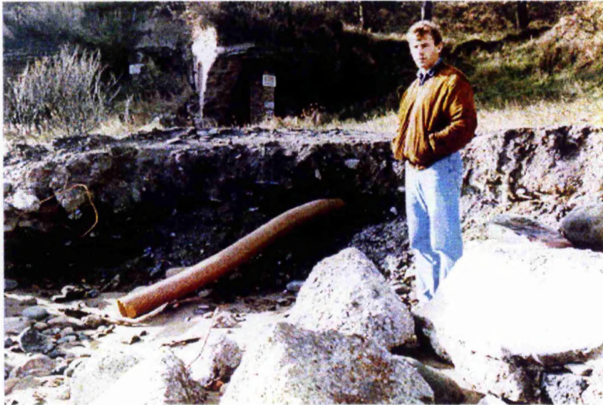
Plate 2.22 East Wemyss Caves, 1993. The orange pipe became exposed by over 2m in less than 6 months and the unconsolidated material around it was being rapidly removed by the sea. The sediment was made up of rubble and colliery waste which was easily washed away at high tide and during severe storms.
