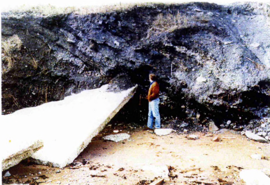
Plate 2.27. The Michael headland in 1993 (the remains of the Michael bing). The slag heap is over 5m in height, and the large concrete slabs have fallen from the upper level of the cliff, showing the extreme instability of this headland.
