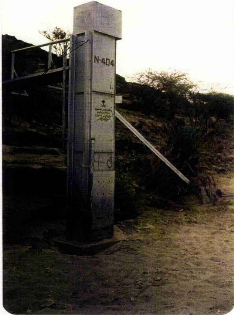
Figure 3.34 Runoff station N-404, Wadi Habawnah-float-type water stage recorders which are generally installed in a shelter house and stilling well.
