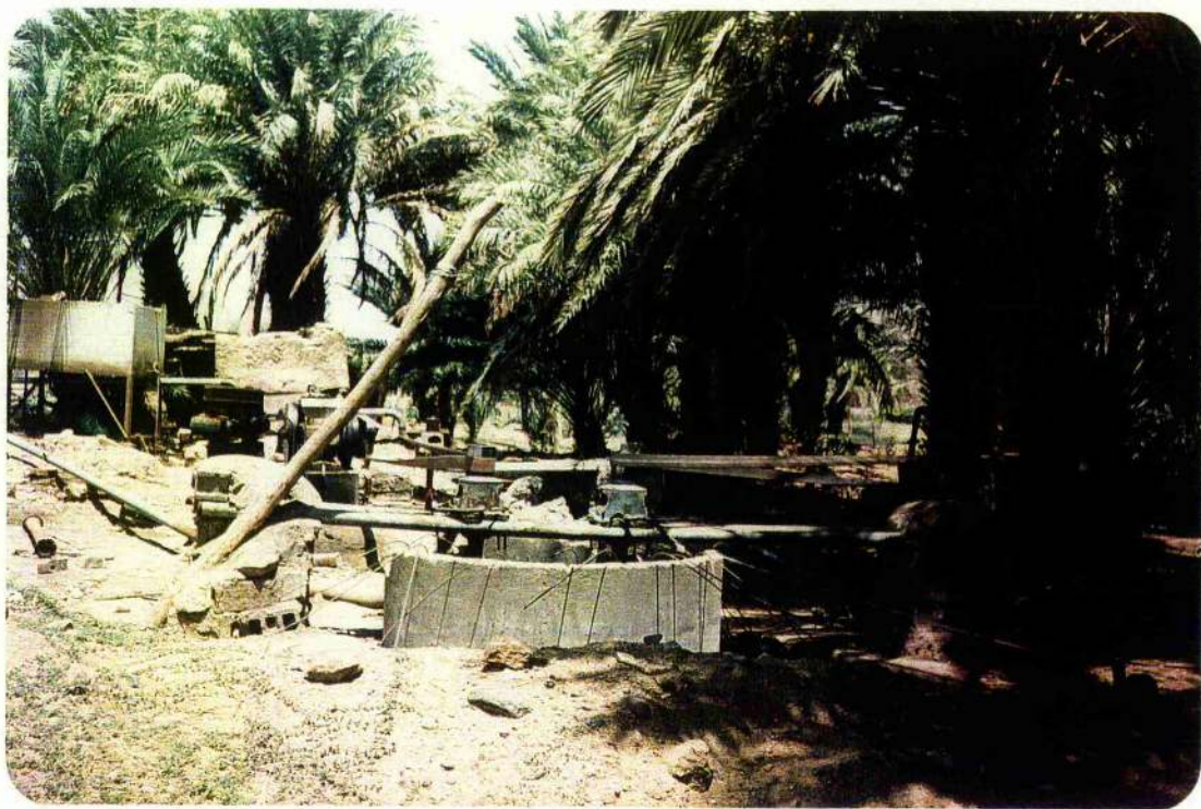
Figure 5.3 Well number MT1 in Wadi Habawnah with concrete lining.
