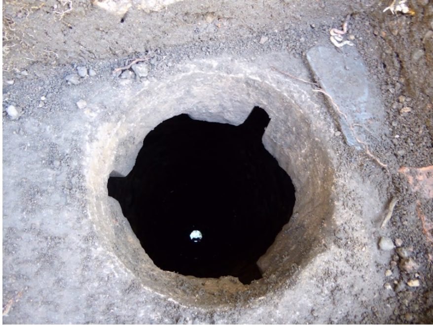
Ph. 1.10.2 © PR The inner part of the covering removed, looking through the old mill-stone to the water.
