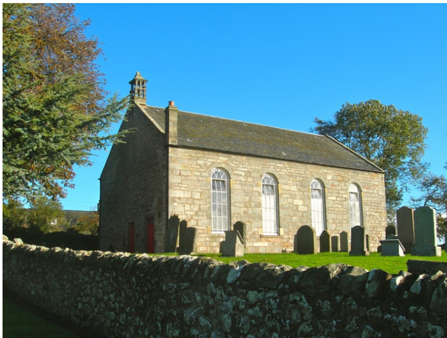
Ph. 2.5 © PR Cameron Parish Church, south facade.
