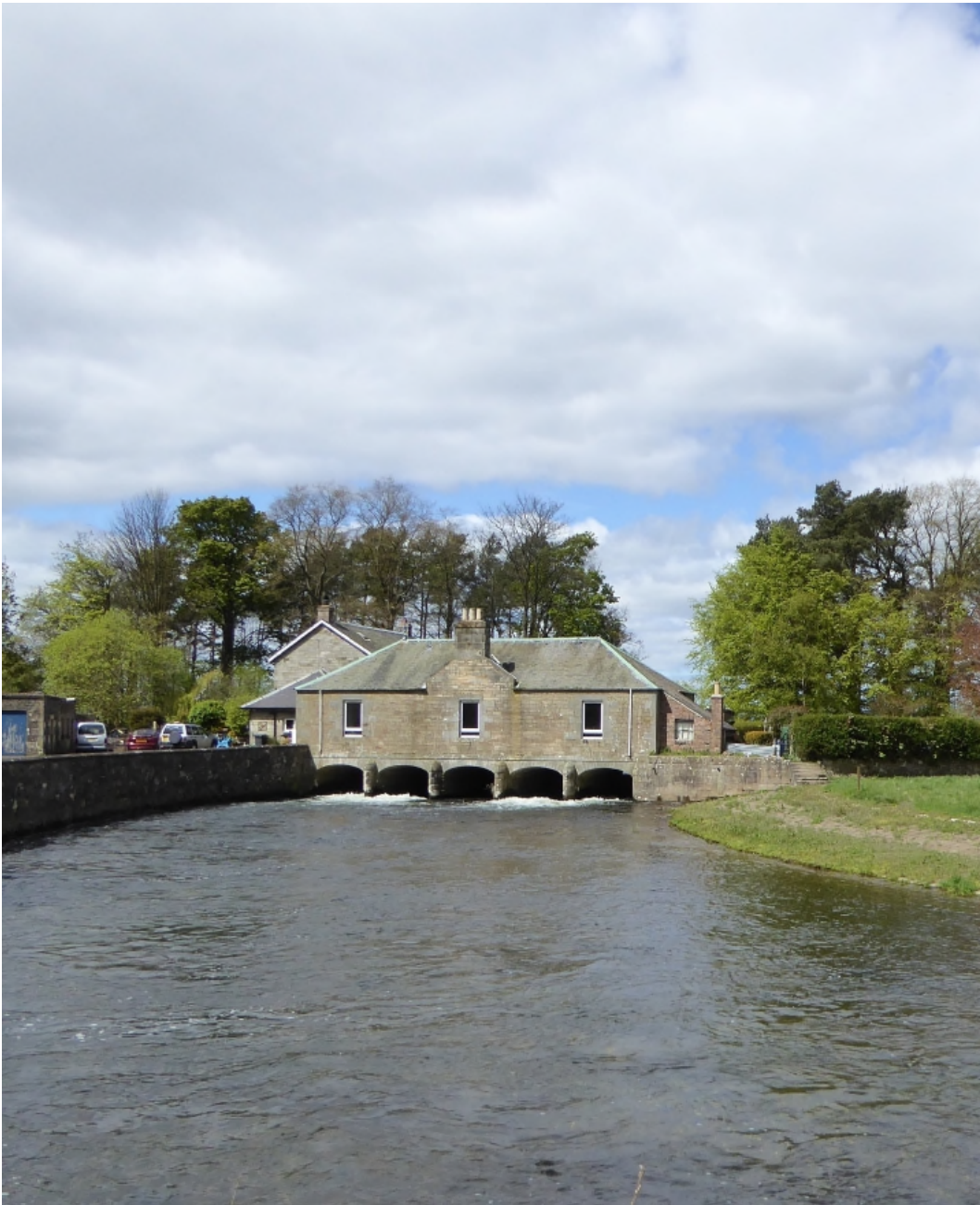
Ph. 2.22 © PR The outfall at the south-east end of Loch Leven, showing the sluices.
