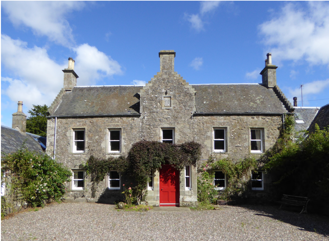
Ph.1.1 © PR Greigston House, south facade.
