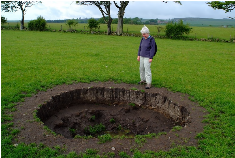
Ph. 1.17 © PR Collapsed access shaft of a bell pit, North Abby field.
