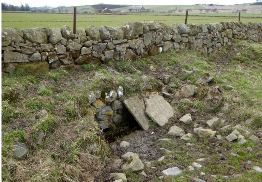
Ph. 1.15 © PR Old drinking trough supplied by piped well water, at the base of a dyke; west side of the field north of East park.
