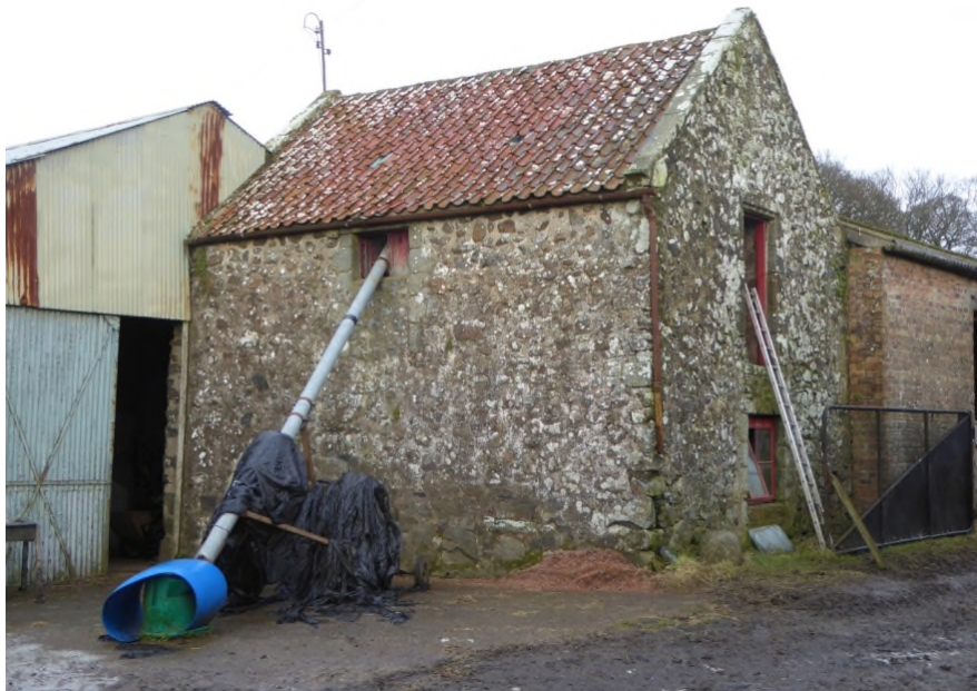
Ph. 1.6.1 © PR The bastle, now part of the steading. The doors indicate the internal upper and lower floors.
