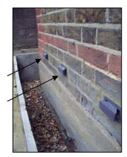
During the rehabilitation, the external ground level adjacent to the house has been lowered by digging a **gravel-filled drainage ditch** deeper than the damp proof course. Rainwater is now diverted in the trench and soaks away via **tubes** pushed deep into the ground below, avoiding the vulnerable wall face.
