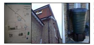
Rainwater harvesting: Several points of capture from rooftop drainage allow extensive rainwater harvesting. The house's different tanks are piped into each other so that overflow from the first storage tank situated in the eaves of the loft extension is captured in a second large tank in a roof space above the property's entrance. The disposition of the tanks allows gravity to deliver
