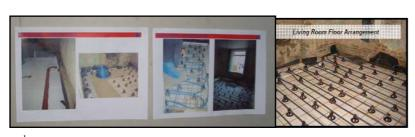
A water-based underfloor heating system, fuelled by the central high-efficiency gascondensing boiler, has been installed throughout the house as it
